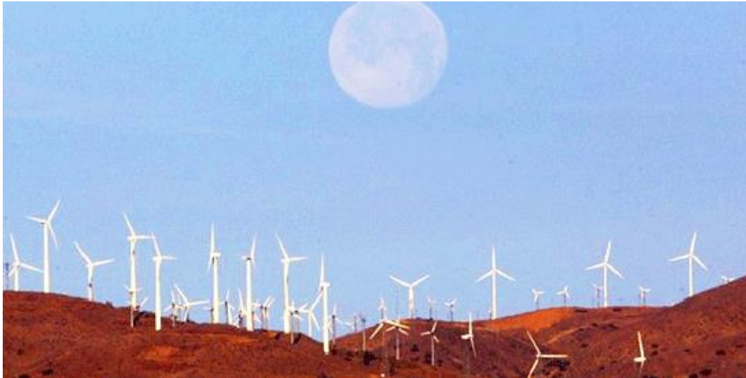
Wind turbines in Jhimpir, Thatta District (Sind)
